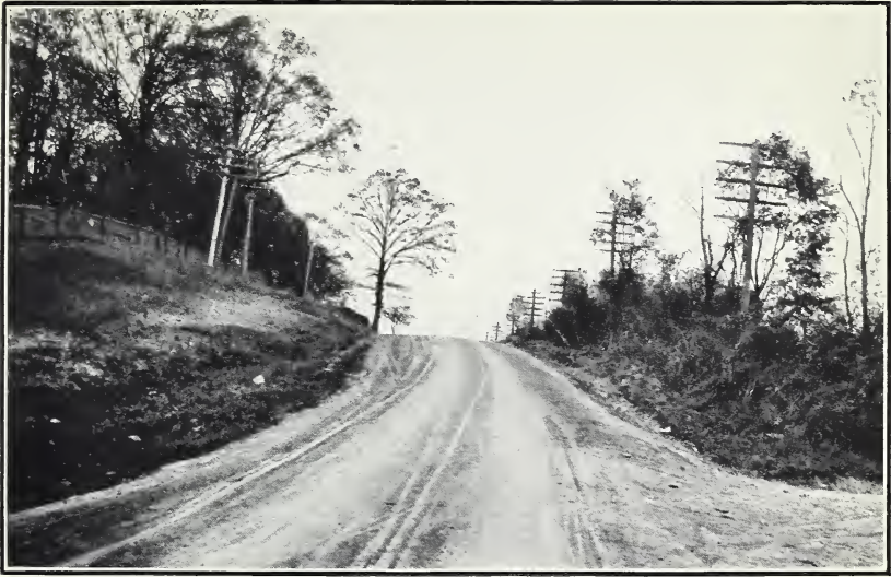
FIG. 1.—GOOD ROAD CROWN MAINTAINED BY DRAGGING, ALEXANDRIA COUNTY, VA.
